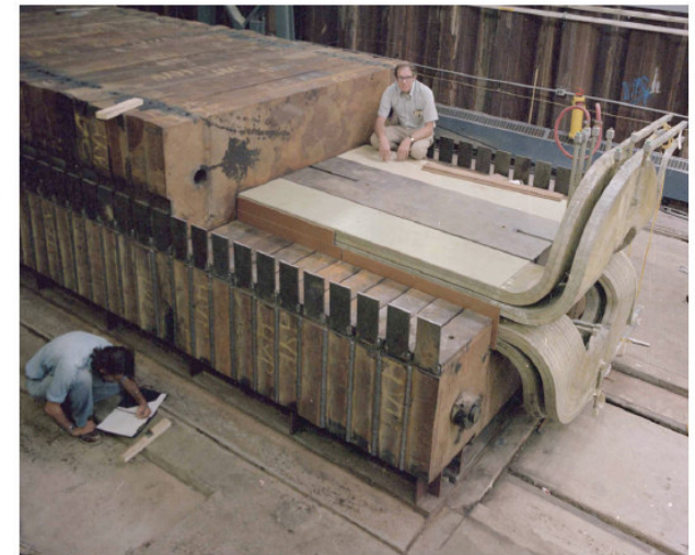
Figure 1 The Hyperon Magnet under construction
