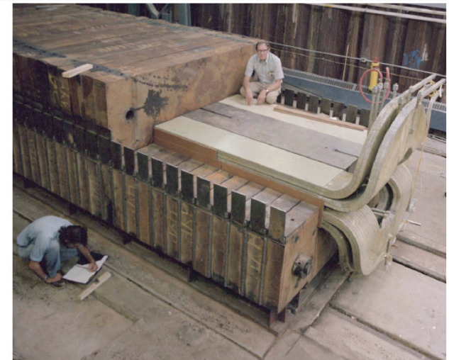
Figure 1 The Hyperon Magnet under construction
