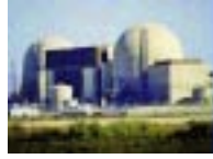
Fig. 14-2. The reactor vessel of a commercial reactor is inside this containment building.
